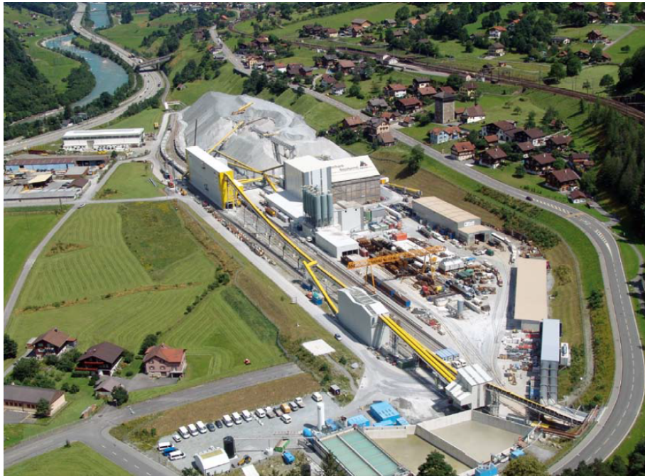
Figure 16: Handling of excavated material at Amsteg, Gotthard base tunnel, close to existing buildings (AlpTransit Gotthard Ltd 2012).
