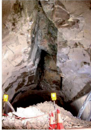
Figure 4. Cave-in section of the fault zone.
