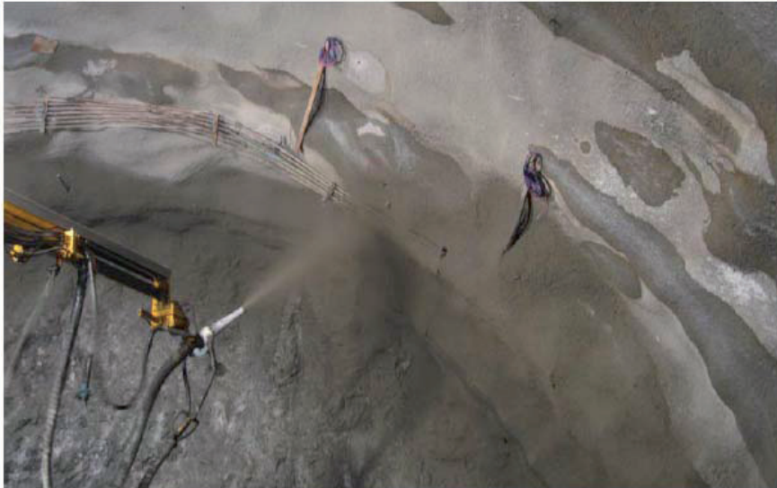
Figure 2.6. Spraying of the instrumented rib (Grimstad et al., 2008).
