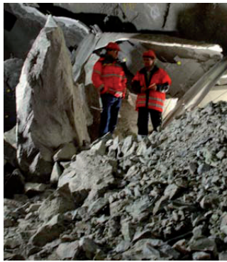
Figure 5. Caved in material.
