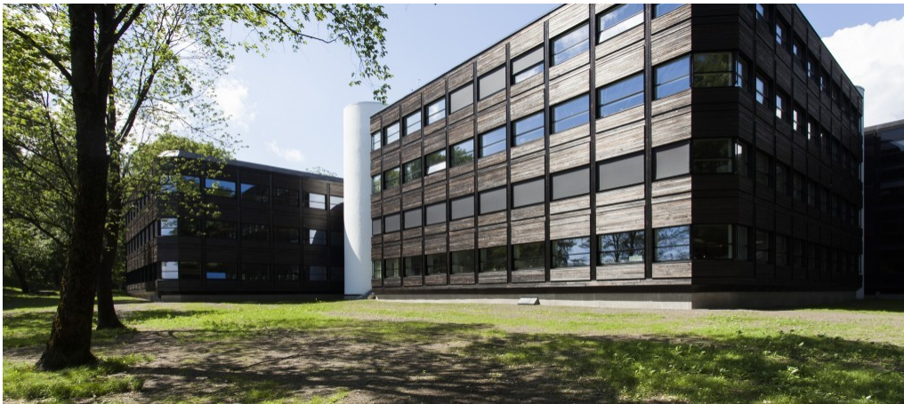
Figure 3.3: Powerhouse Kjørbo from the outside. Left is Block 5 and right is Block 4. Photo: Powerhouse Alliance.
