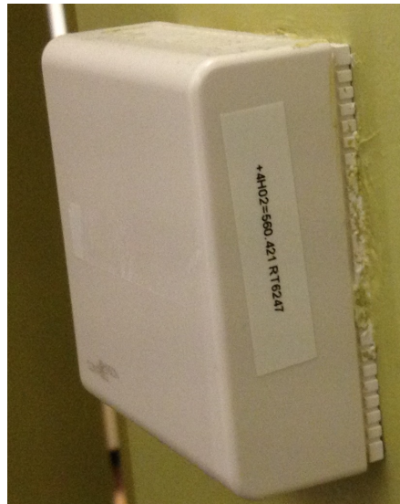
Figure A.2: The A99RY-1C temperature sensor at Powerhouse Kjørbo. Photo: Odin Søgne.
