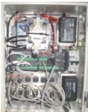
Figure 4–16: Left: Logging cabinet with a data logger placed in the manhole around the top of borehole 3 at Bryn. A GSM-module makes remote-controlled monitoring possible. Right: The control panel for the pilot plant at Bryn consists of motor protections for the pumps and a flood shelter for the manhole.
