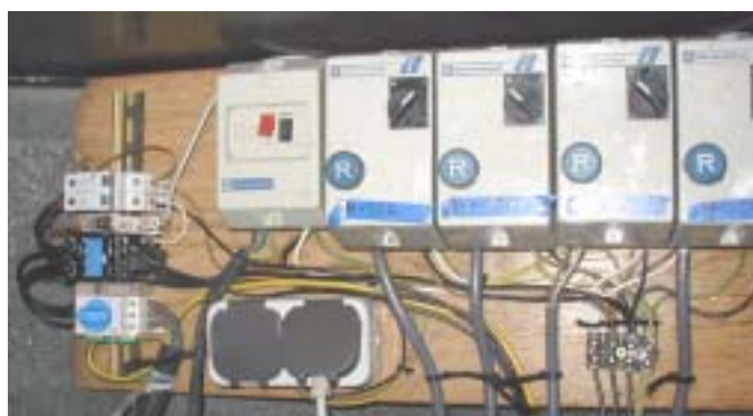
Figure 4–16: Left: Logging cabinet with a data logger placed in the manhole around the top of borehole 3 at Bryn. A GSM-module makes remote-controlled monitoring possible. Right: The control panel for the pilot plant at Bryn consists of motor protections for the pumps and a flood shelter for the manhole.
