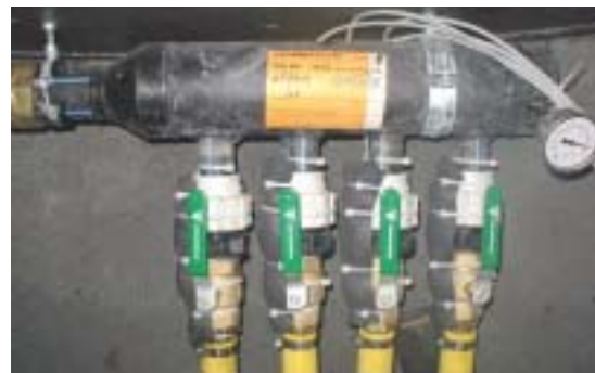
Figure 4–15: Left: The flowmeter and the heat exchanger in the manhole around the top of borehole 3 at Bryn. Right: Manifold collecting the pumped groundwater from the satellite boreholes. The system pressure is monitored by an analog manometer. Temperature sensors were fastened with isolation material and plastic bands.
