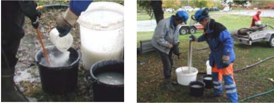
Figure 4–17: Mixing of water, guar gum (thickener) and sand. Filling of injection fluid into the high-pressure tank is shown in the upper right corner.
