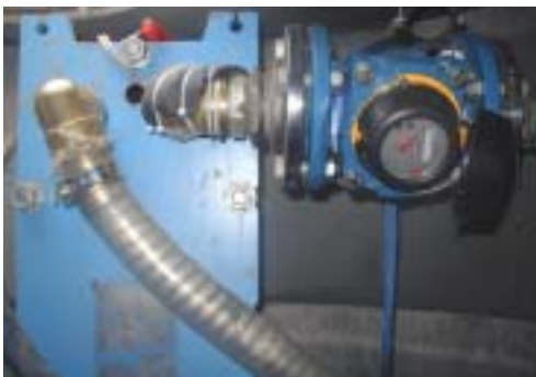
Figure 4–15: Left: The flowmeter and the heat exchanger in the manhole around the top of borehole 3 at Bryn. Right: Manifold collecting the pumped groundwater from the satellite boreholes. The system pressure is monitored by an analog manometer. Temperature sensors were fastened with isolation material and plastic bands.
