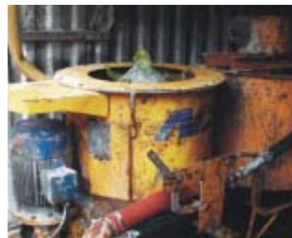
Figure 4-6: Mixer, container and injection pump.
