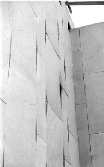
Figure 1. Bowing of marble claddings (from TEAM brochure, see also www.sp.se/Building/TEAM )
