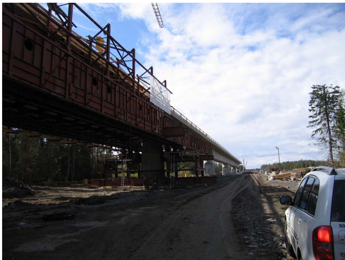
Figure 19 A concrete beam railway bridge under construction. The slipform is shown in the foreground and the finished bridge is shown in the background.
