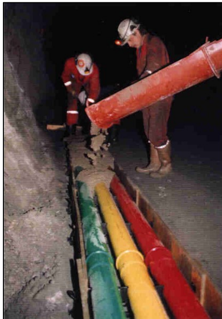
Figure 3-14: Burying current cables in the ground of tunnel (Egil 2013a)
