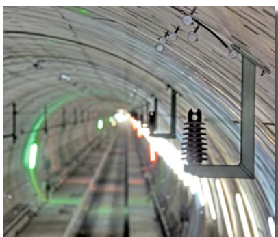
Support point with reinforcing conductor with connection to the return conductor
