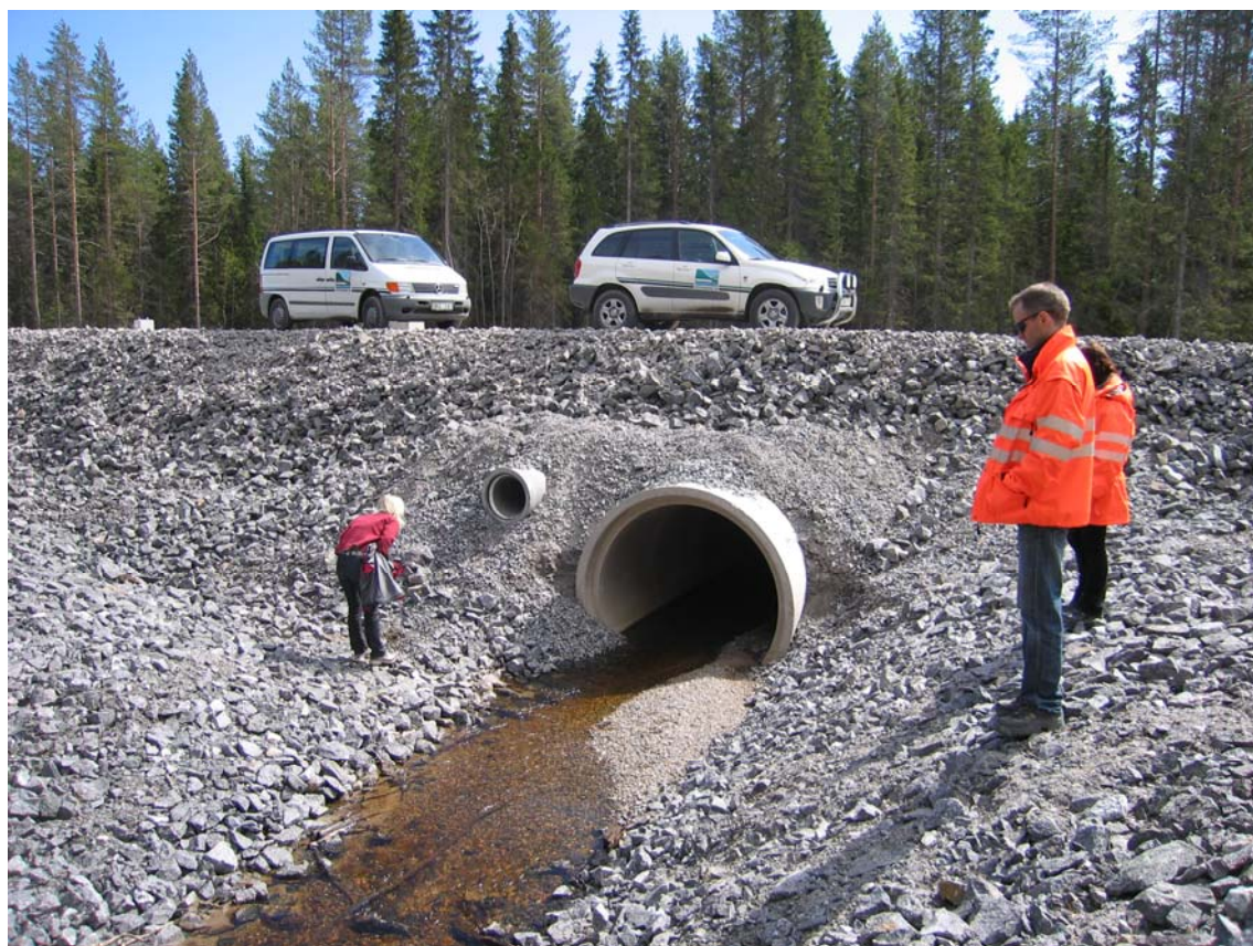
Figure 8 Culverts are needed in the track foundation for water and wildlife. The picture shows a culvert for a water course (large) and a separate, dry wildlife passage (small).
