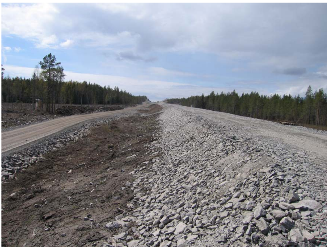
Figure 7 To the right, a typical railway track foundation. The service road parallel to the railway is shown to the left.
