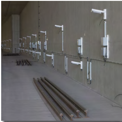
Installation work Safety lighting
