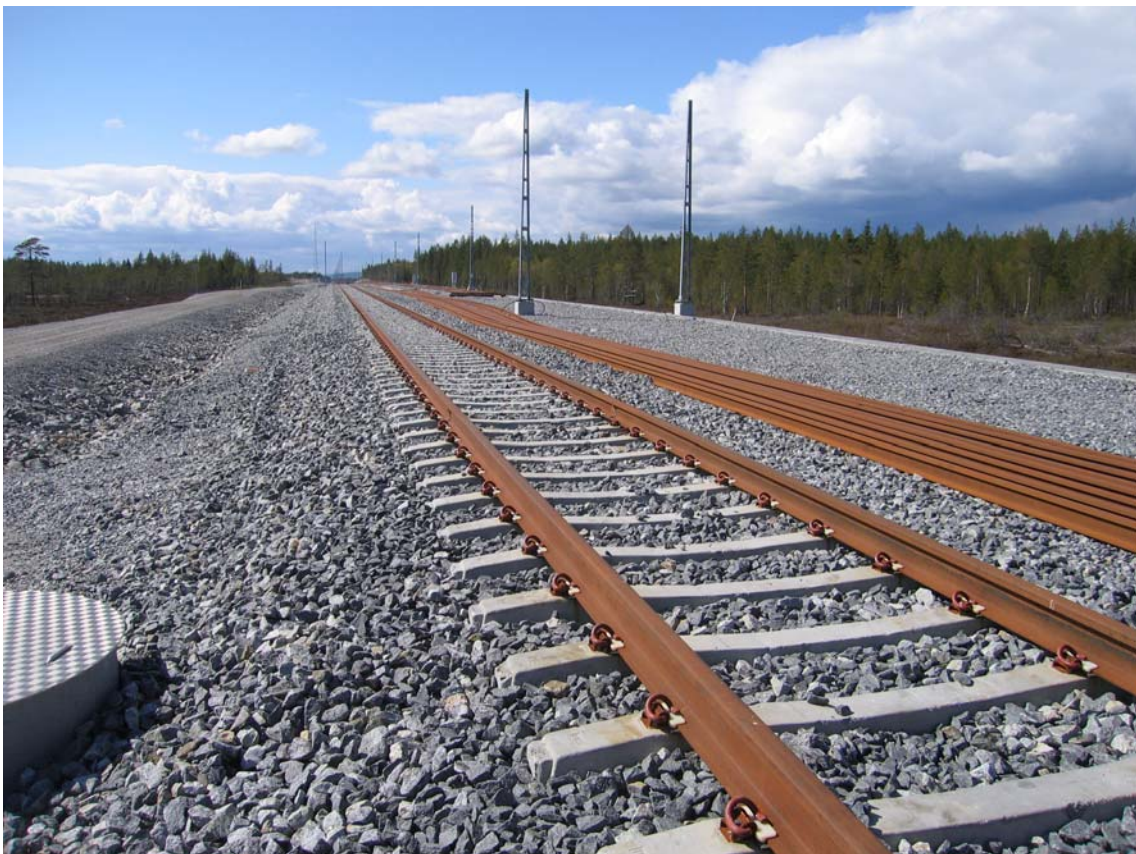
Figure 10 The picture shows a typical railway track with rails attached to concrete sleepers with rail fastening. The space between sleepers are filled with track ballast.
