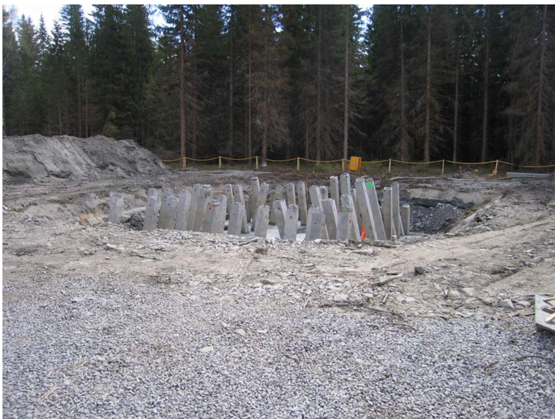
Figure 20 The picture shows an example of foundation work for a bridge pier. In this case, the ground has been excavated, stabilized by precast concrete piles and a concrete foundation has been cast.
