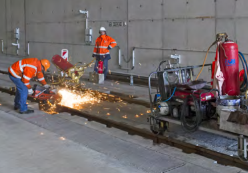
Installation of modular and long-welded rails
