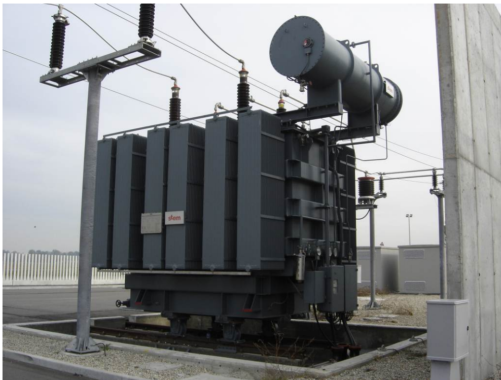
Figure 4 Power transformer 60 MVA at Fissiraga traction substation at high speed Milan – Bologna section (Source: Rete Ferroviaria Italiana)
