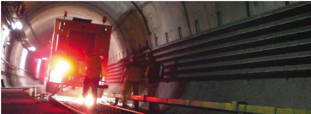
Figure 10 Rail Grinding in Vienna's metro system (Source: Wiener Linien)
