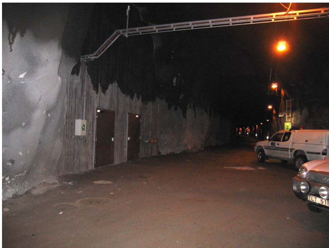
Figure 16 Example of a service tunnel. The doors are a part of the evacuation lock from the main tunnel to the service tunnel.
