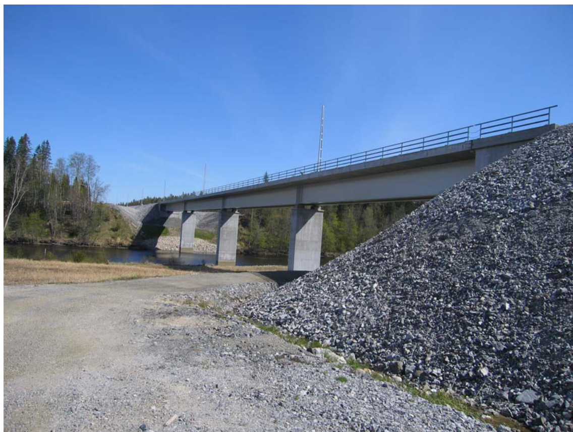
Figure 18 A steel girder railway bridge. To the right in the picture, the erosion protection of the slope is shown.
