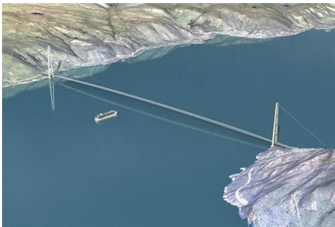
Figure 9: Overview of the 3700 meter single span suspension bridge Illustration by Statens vegvesen
