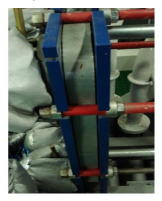
Figure 83: LNG Evaporator Circuit Heat Exchanger
