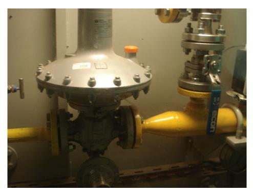
Figure 5: Gas Ramp Unit (GRU)
