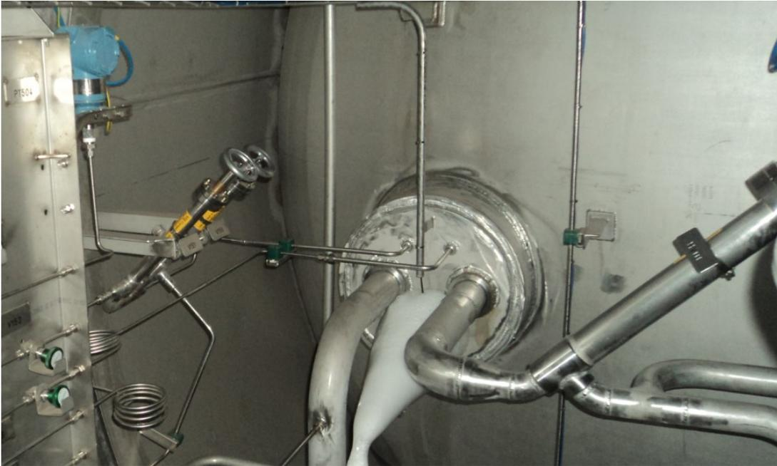
Figure 45: Trycock piping in the Cold Box on MF Korsfjord
