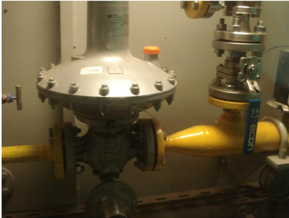
Figure 5: Gas Ramp Unit (GRU)
