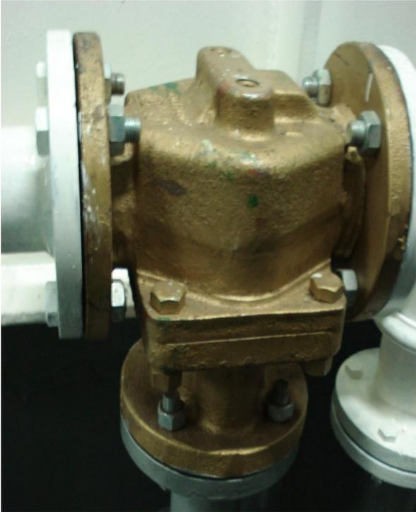
Figure 82: Amot Thermo-Mechanical Valve
