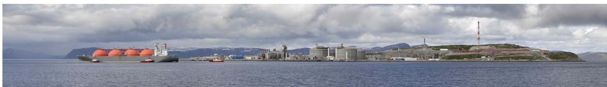
Figure 5.2.2: Melkøya LNG plant and export facility, Wikimedia Commons
