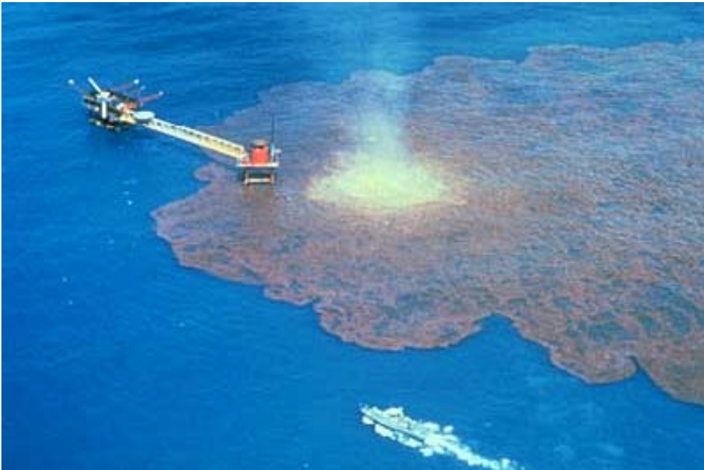
Figure 1.2.: The result of a blowout[Services, 2004]
