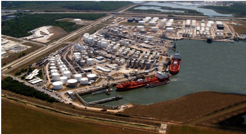
Figure 2.4: A terminal where chemical liquids can be loaded or unloaded (Odfjell, 2015)
