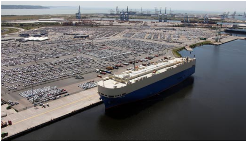
Figure 11.1 – RoRo terminal facilities in Le Havre, France. Source: Grand Port Maritime du Havre
