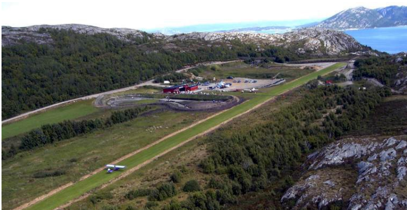
Figure 7.1: Aerial photo of Agdenes Airfield. Image courtesy of norskeflyplasser.no .
