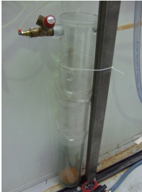
Figure 3.5: The air buffer tank.
