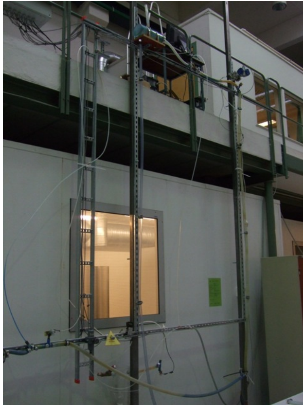
Figure 3.3: Overview of the Mini-loop experiment. The inlet is in the lower left corner. The riser starts in the lower right corner and goes up to the upper right corner. On the horizontal top section, the DP-cell, pressure sensor and choke valve are installed. The separator is located in top after the horizontal top section.
