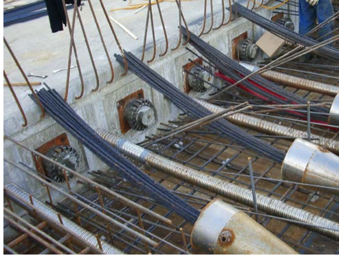
Figure 16 Example of preparation of couplers R with strands. [20]
