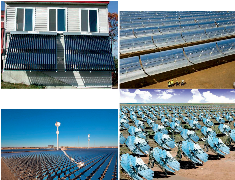
Figure 1.3.: Domestic hot water solar heater, CSP power plant with parabolic troughs, solar tower with heliostats, and paraboloids with Stirling engines [12]
