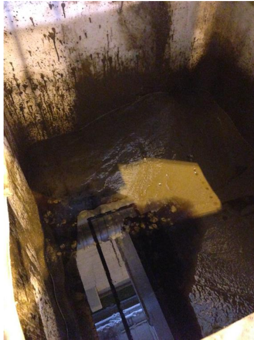
Figure 34: Tank for sand that is filtered out from the flow loop
