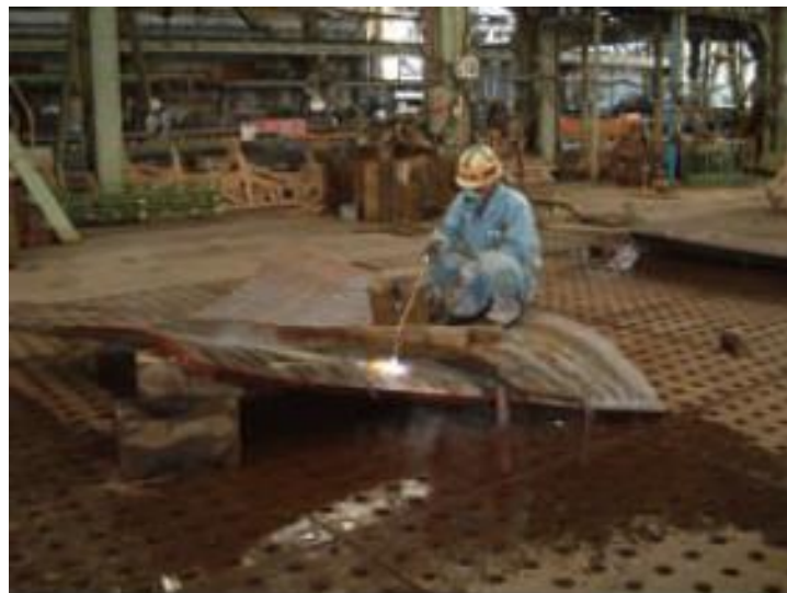
Figure 14 - Manual heat-line work, bending steel plates. Source: (Yoshihiko, 2011).
