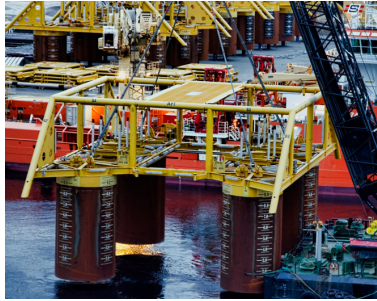
(a) A typical suction anchor (EniNorge, 2014)
