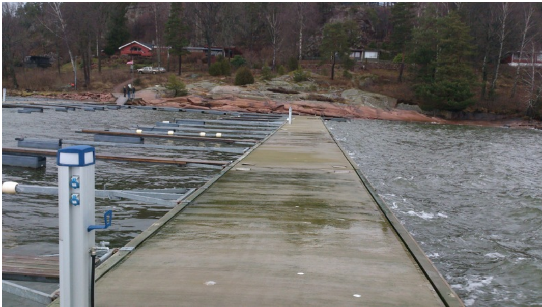
Figure 3.4: Hinged outriggers PHOTO: Bi-Brygga AS
