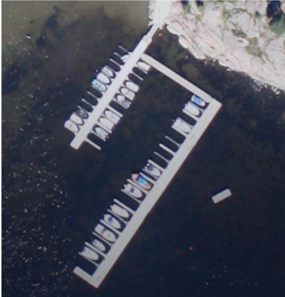
Figure 3.1: Floating dock system in Sande, Vestfold. PHOTO: NORKART AS
