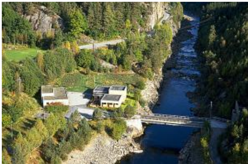
Figure 5-2 Laudal power plant. Extracted from Agder Energy web page.
