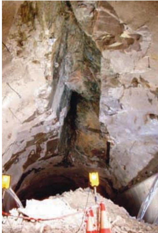
Figure 3. 2: Example of block downfall from structurally controlled instability. From the Hanekleiva tunnel, Norway (Beitnes et al., 2007).
