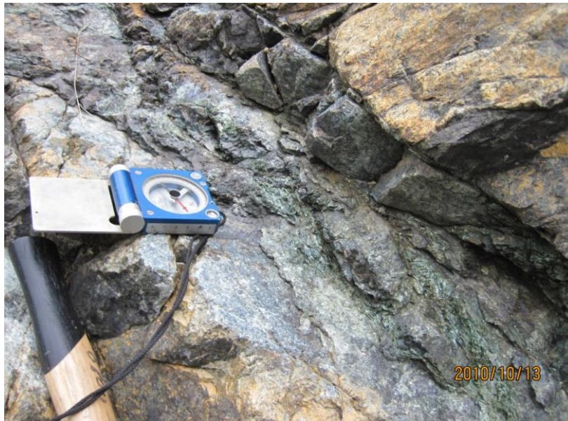
Figure 4. 8: Weakness zone within the rocks of the Devoll ophiolite massif along the state road, dm-scale, filled with serpentine minerals (DHP, 2011)
