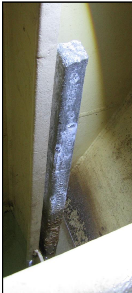
Figure 11: Two meter long zinc anode on KV Bergen
