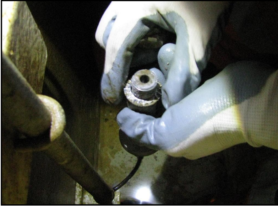
Figure 32: The Membrane has been Prone to Fouling
