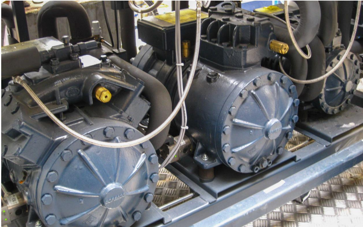
Figure 5.4: The rack of the piston-type R744 compressors. On the left: base-load Dorin CD1400H, parallel #1 Dorin CD1000H, and parallel #2 Dorin CD380H.
