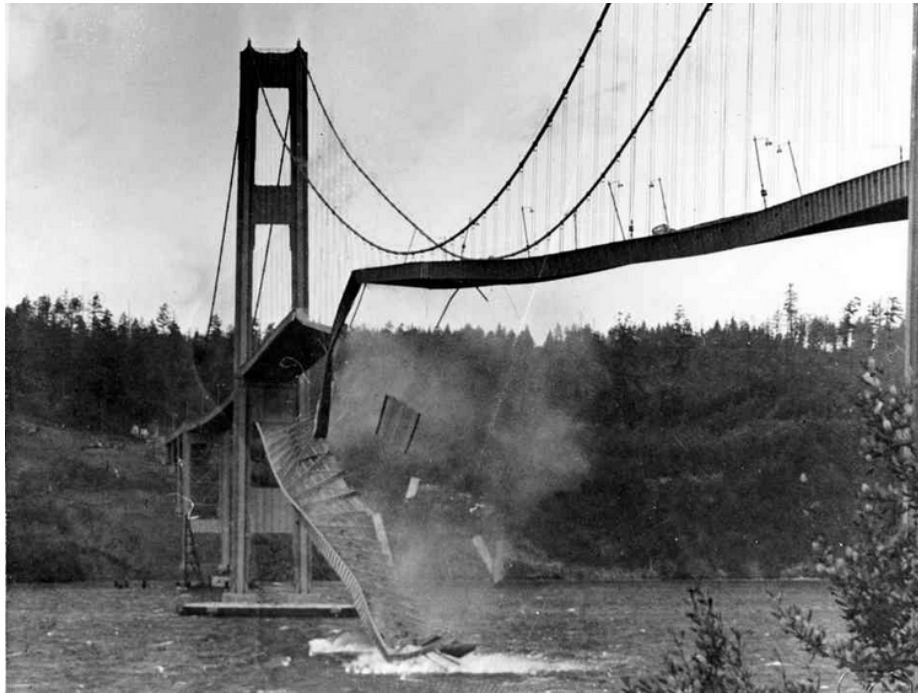
Figure 3: The Tahoma bridge in Washington, USA was brought down by wind gusts with the same frequency as the bridge natural frequency only months after opening [7].
