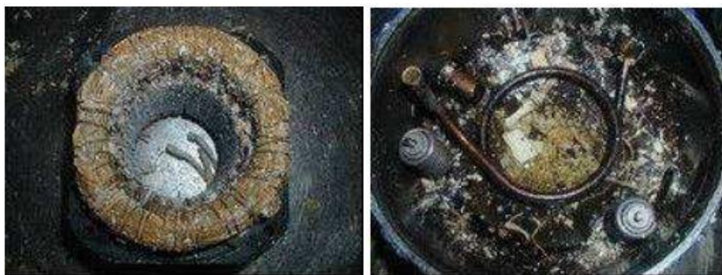
Figure 13 LT- 28-4VI compressor after breakdown (Danish Technological Institute, 2005)
