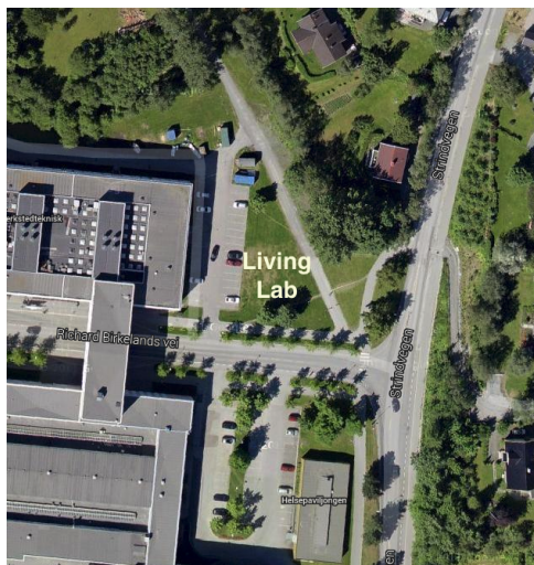
Figure 21: Real building site (GoogleMaps, 2015).
