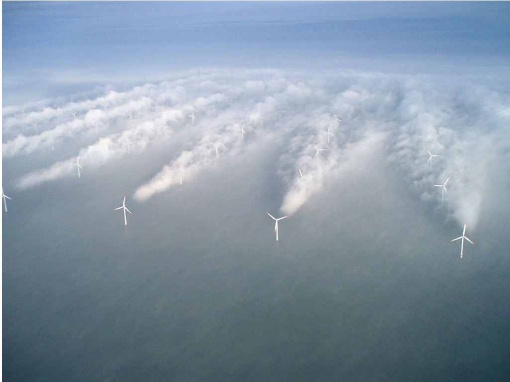
Fig. 8. Wake turbulence behind wind turbines – photo of Horns Rev offshore wind farm in Denmark [21].
