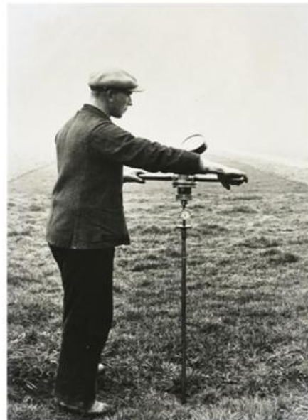
Figure 1.1 The first manual CPT apparatus
