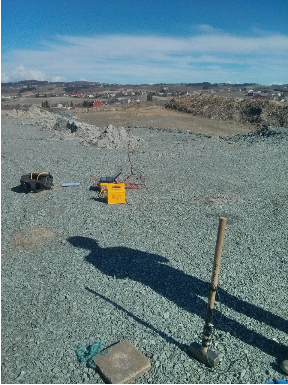
Figure 4.11 MASW setup at Klerr (Photo: Eide, H)
