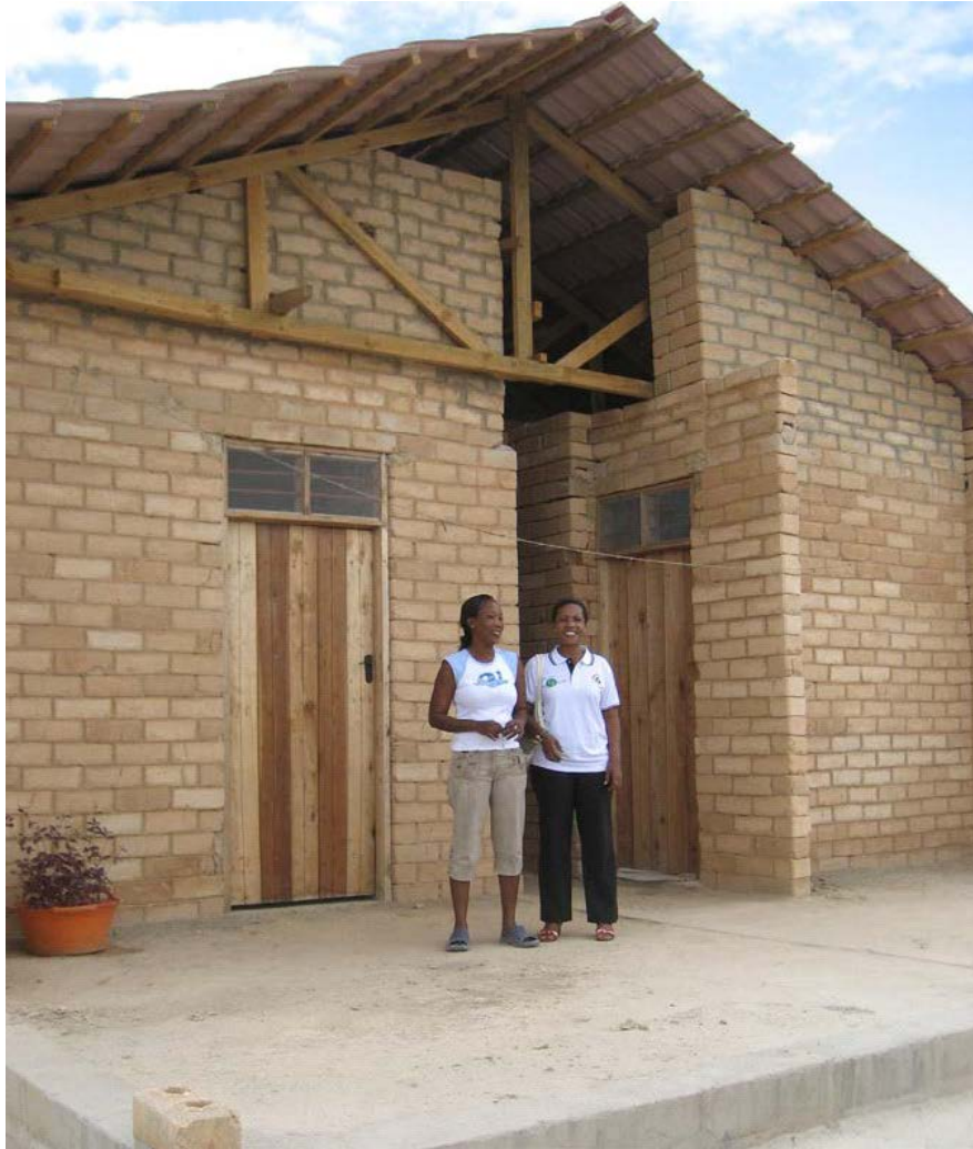
Figure 4.3: A partly built house in Chamazi, photo by: Margaret Ricke, 2011
