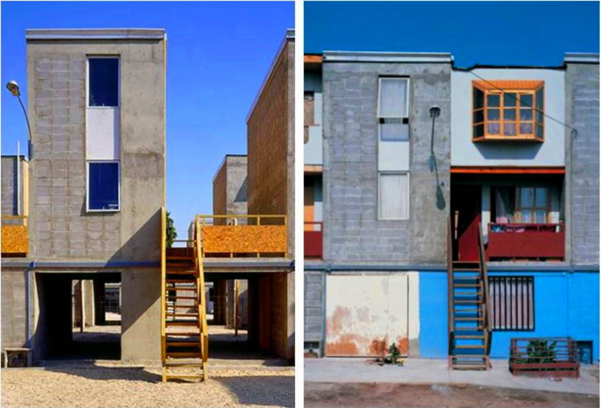
Figure 2.12: Left: Quinta Monroy as it appeared when construction was complete. Right: Quinta Monroy after self-construction. Source: Elemental
