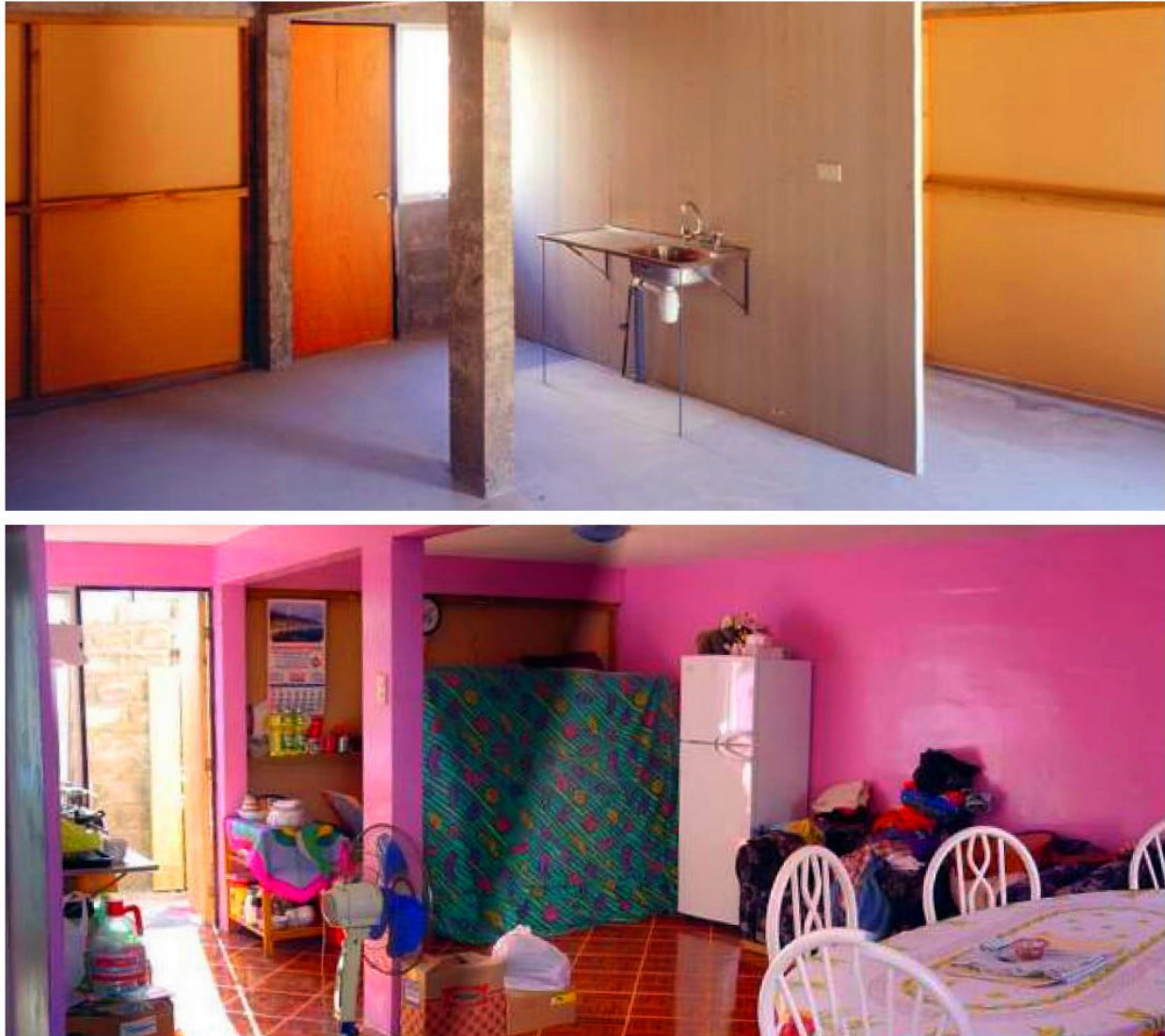
Figure 2.13: Interior views of a unit in Quinta Monroy showing before (up) and after (down). Self-constructed modifications include windows, floor surfaces, and painting. Source: Elemental
