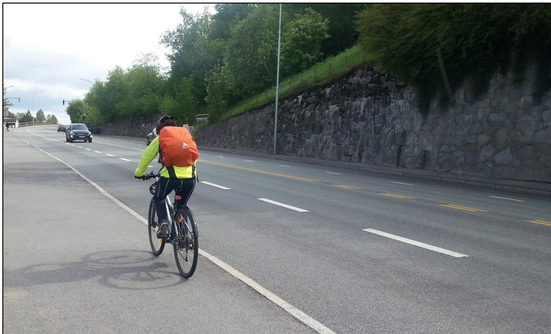
Figure 1: Photo of the current road
