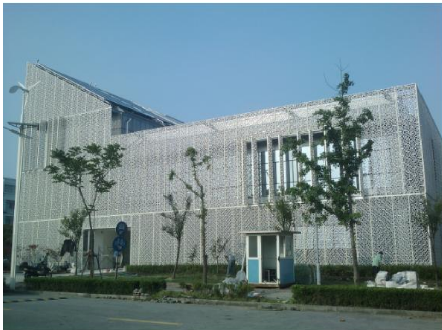
Figure 18: The GEL-building located in Shanghai Jiao Tong University
