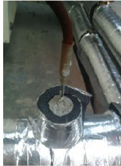
Figure 41: PT100 sensor covered by a silicon substance
