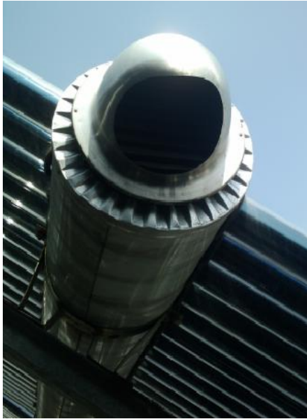
Figure 29: Entering point of the regeneration air
