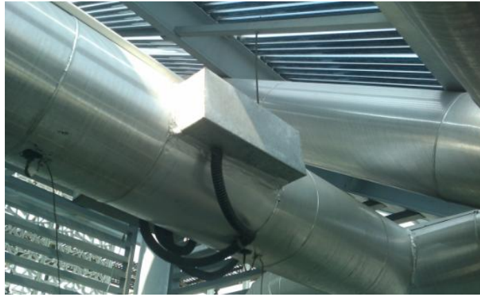
Figure 31: The auxiliary heater of the system, 3 kW, 6 kW and 9 kW
