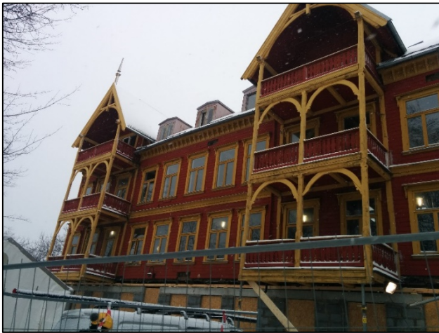
Figure 5: Thingvallagården – Main building - 2015
