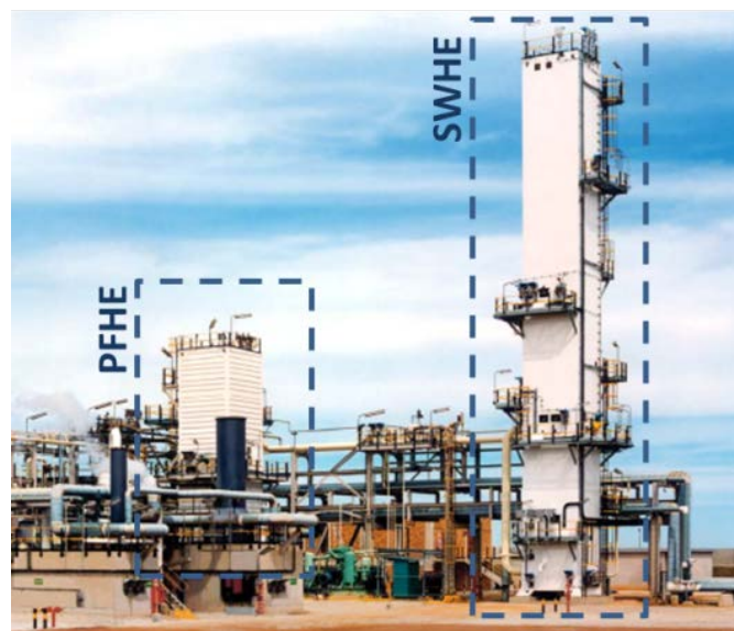
Figure 2-23. Compactness of spiral wound heat exchanger versus plate fin heat exchanger [40]
