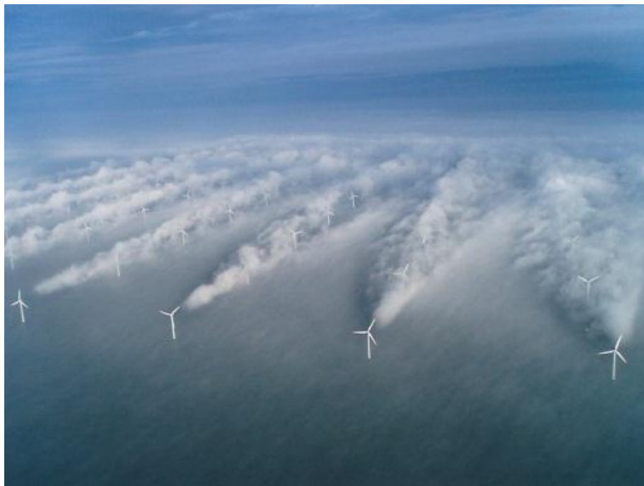
Fig. 1.8: Wind turbine wake effects in the Danish offshore wind farm “Horns Rev 1” [20]
