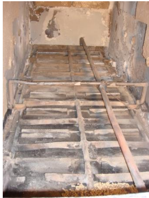
L.4 Ash after combustion with 8 percent sewage sludge
