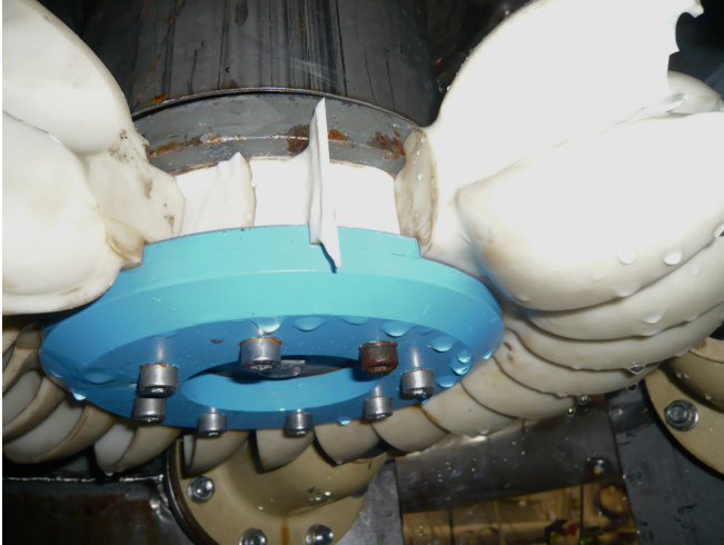
Figure E.5: The turbine in place in the turbine housing after the failure
