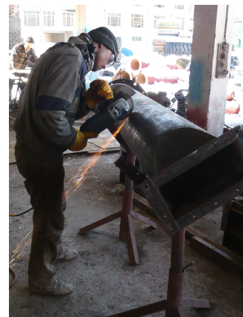
(e) Pipe cutting
