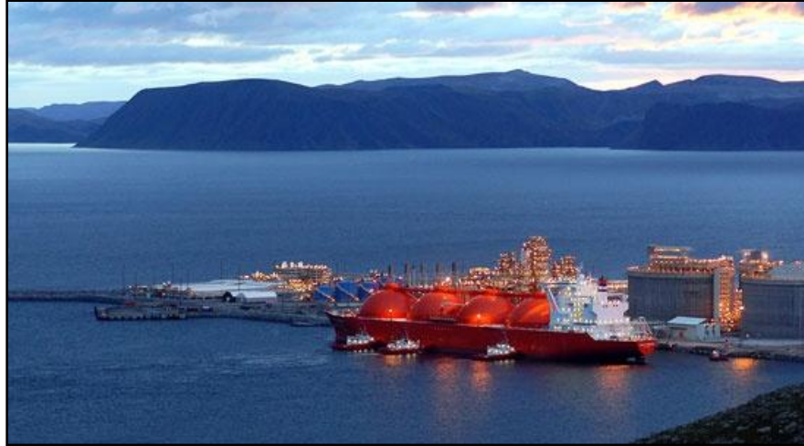
Figure 2.1: The processing plant at Melkøya. Image courtesy of StatoilHydro
