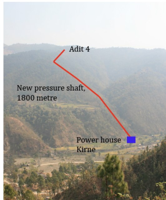
Figure 3.3: The new pressure shaft of Kirne Power Plant, as it is planned.
