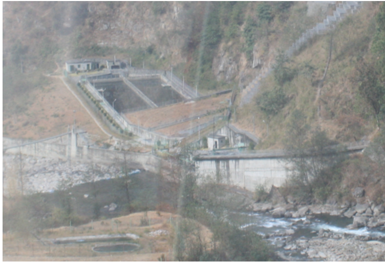
Figure 2.14: The intake seen from helicopter.
