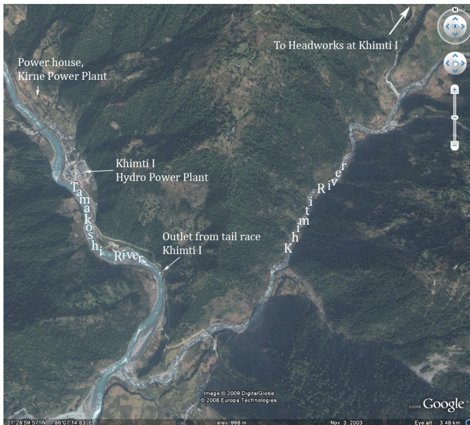
Figure 1.3: Air photo over Khimti I and the junction between Khimti Khola and Tamakoshi Khola. Different places and items are marked on the photo. Taken from Google Earth 19.01.2009. [25]
