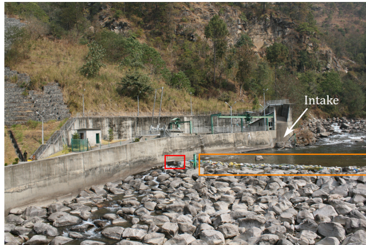
Figure 2.13: The intake at Khimti I/Kirne Power Plant
