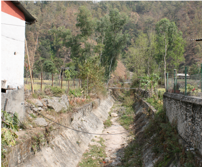
Figure 3.5: The planned outlet from Kirne, through the existing canal shown.
