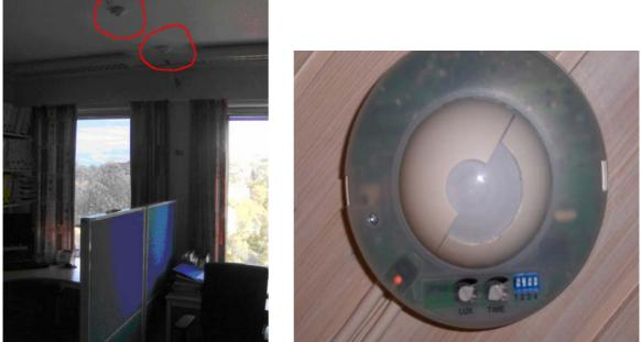
Picture 3. Left; Typical office room fitted with two ceiling-mounted sensors. Closest sensor is a SWE sensor and the other is a MIM sensor.
