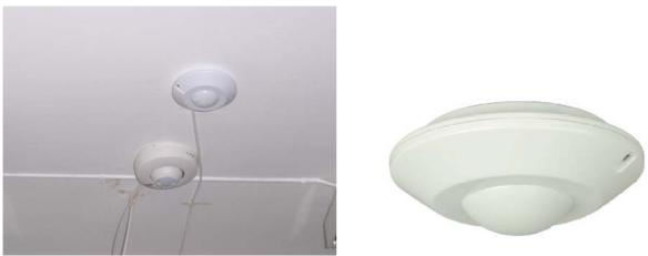
Picture 7. Left; Typical mounting of the SWE and MIM sensors. Picture 8. Right; SWE sensor. Same as the top sensor in Picture 7.
