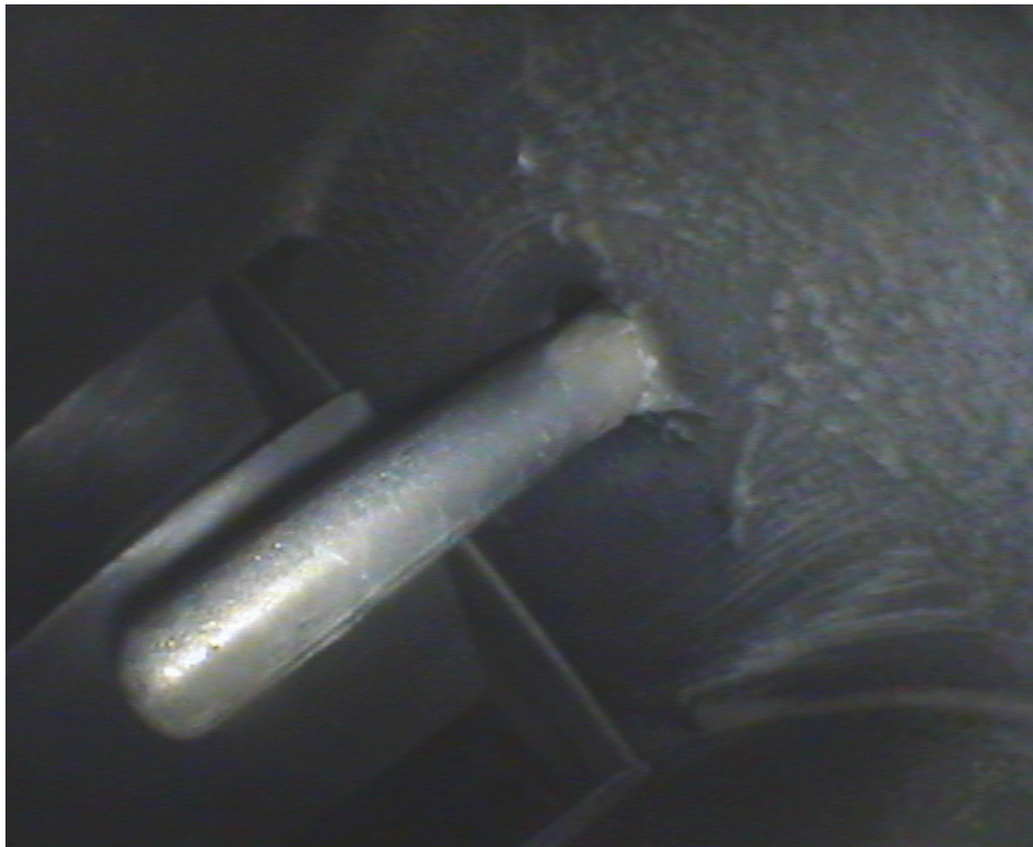
Figure 30 Salt deposits on first stage temperature sensor
