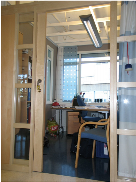
Figure 6-8 Room with the suspended ceiling removed (EC)
