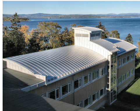
Figure 2 The TKS wing viewed from south-east, showing the air exhaust tower and the glazed staircase.
