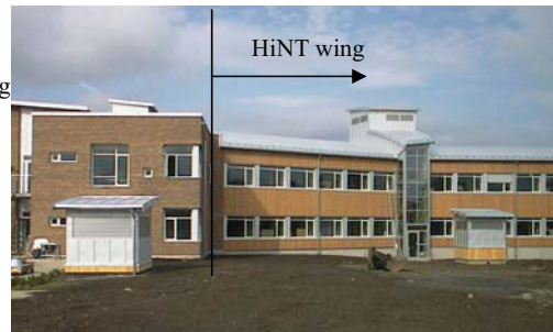
Figure 2. The east façade with the air intake towers in the foreground. The right tower supplies the office wing. The glazed area is the stairwell. The tower above the stairwell is the exhaust air tower.
