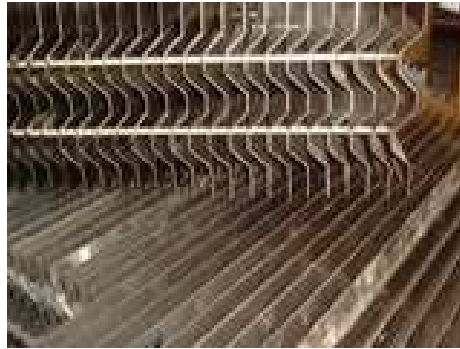
Figure 1.6: Details of a vane pack demister [158]
