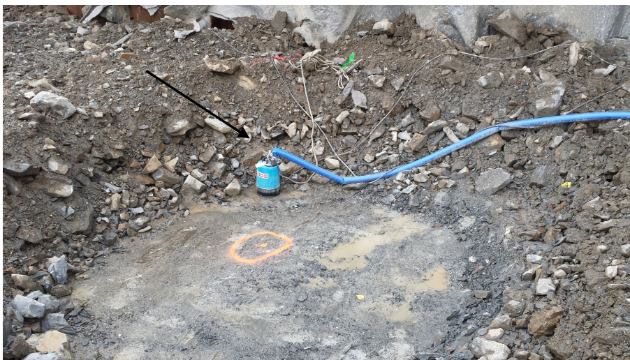
Figur 2.34: Pumpe for overflatevann
