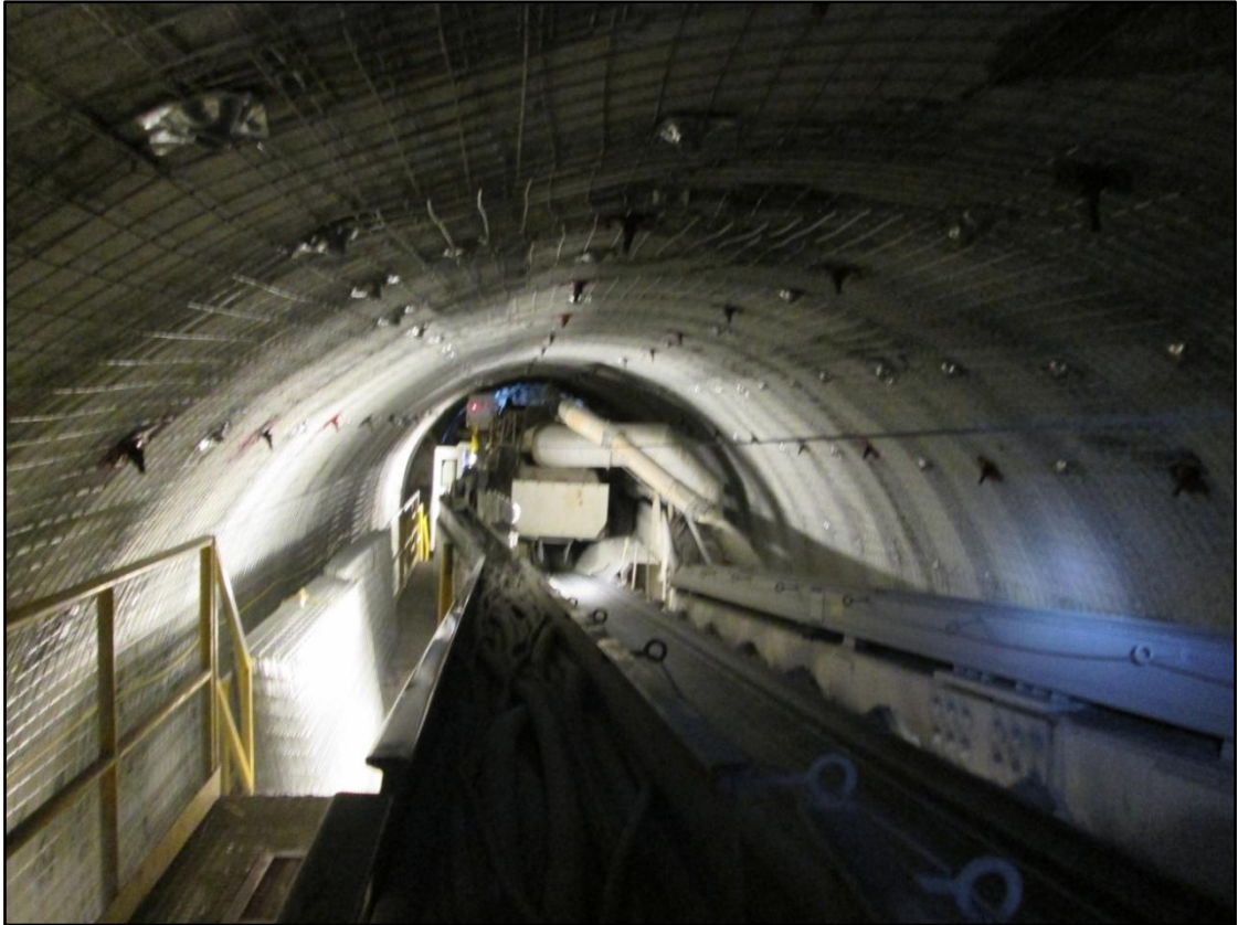
Figure 3.3: Tunnel profile with installed rock support
