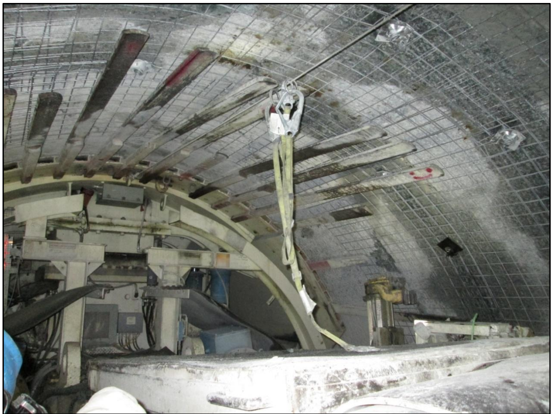
Figure 3.4: Area behind the TBM cutterhead
