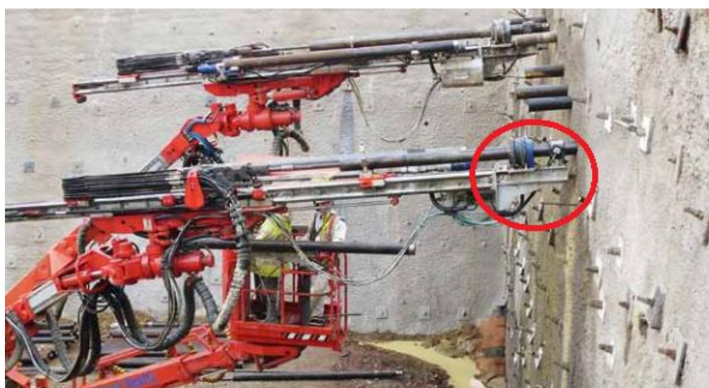
Figur 5-10: AT- Pipe Umbrella Automation Unit er markert. (Dywidag-Systems, 2013)
