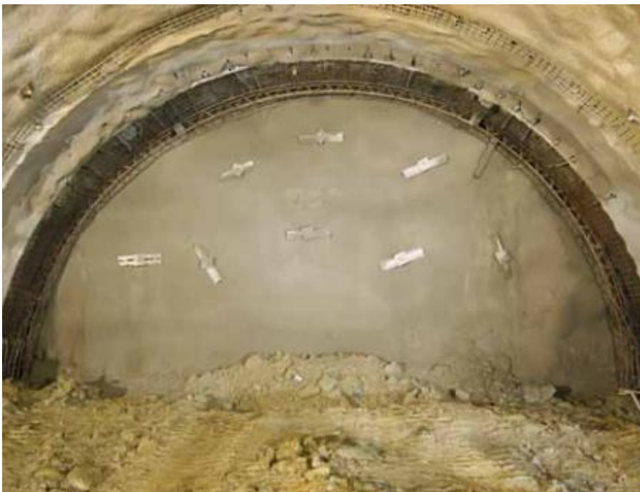
Figur 5-22: Pantex gitterbue sett inn mot stoff. (HWE, 2014)
