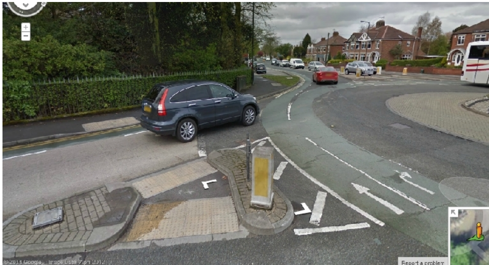
Fig. 15. – Continental-style roundabout with cycle lanes at Heworth Green in York, UK
