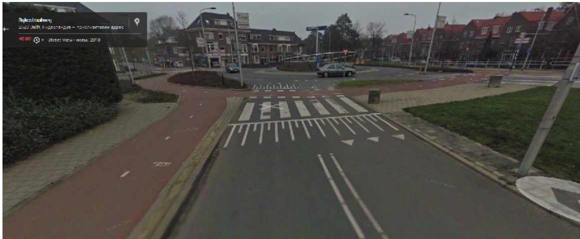
Fig. 74. Roundabout with a raised crossing in Delft, The Netherlands
