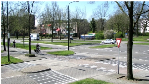
Fig. 9. – Well marked, reddish colored, raised bicycle crossing 9
